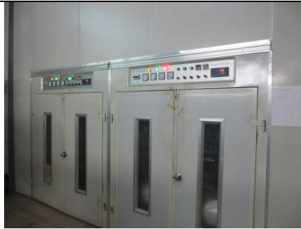
Slaking workshop 熟化车间
